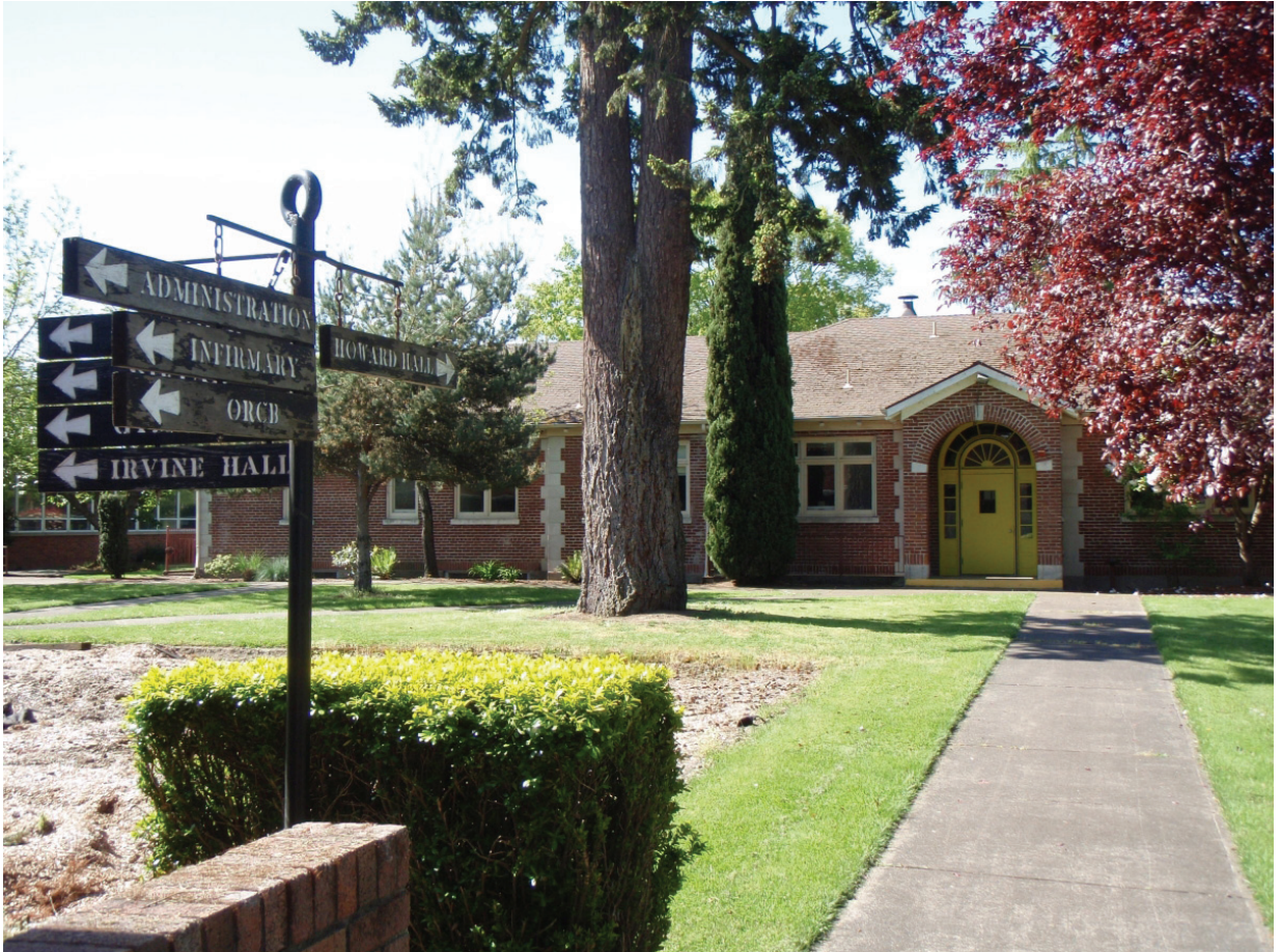
Howard Hall North Elevation
