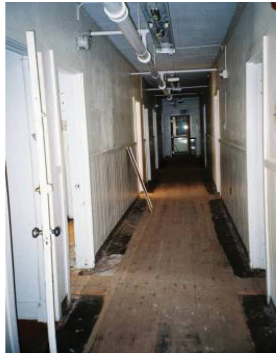
Asbestos and lead paint abatement work was completed in 2012.
